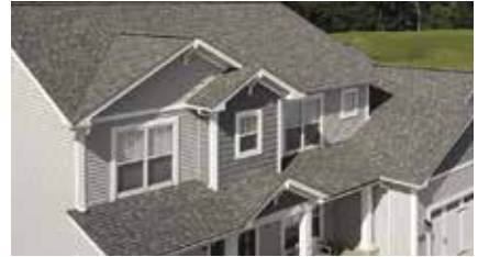
ROOFING AND VENTILATION
